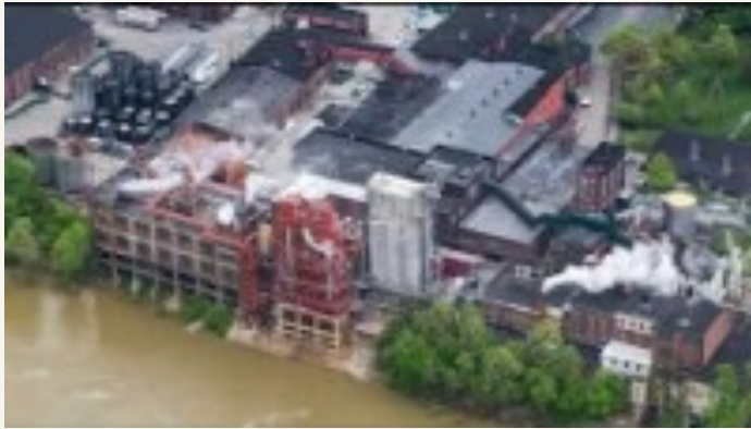
Buffalo Trace Distillery Expansion
